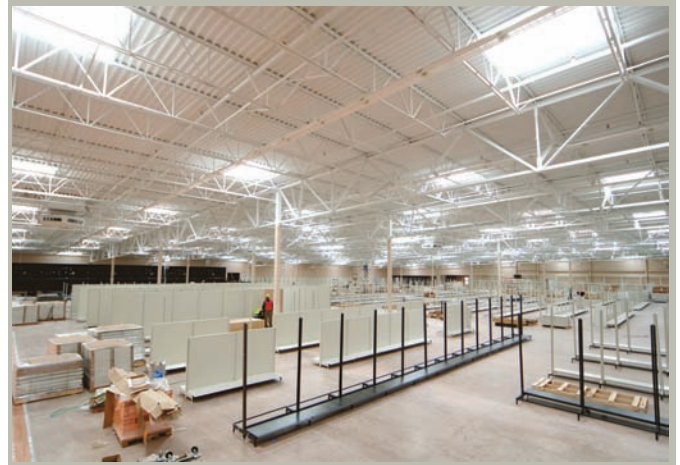
Interior painted, skylights installed, and NO ELECTRIC LIGHTS ON. Prismatic skylights produce the highest visible light transmittance with 100% diffusion. Net result, even light without the undesirable hot spots.
