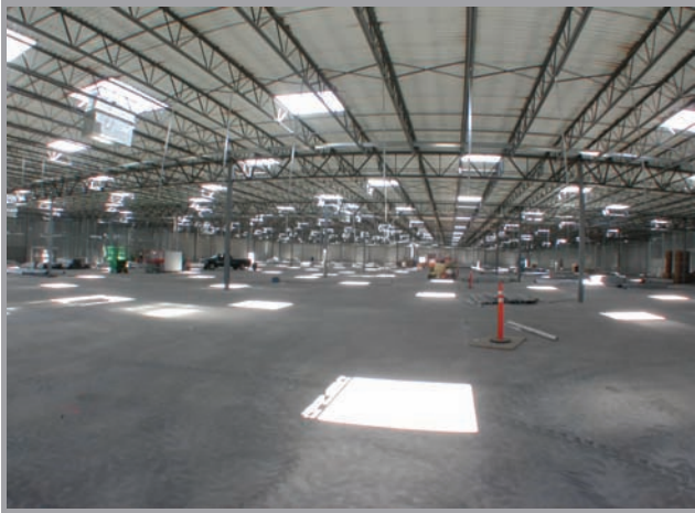
Walmart Supercenter under construction. Skylight openings in place, steel deck roof and steel trusses ready for white paint. Direct sun hot spots abound similar to the effect found in systems with clear glazings.
